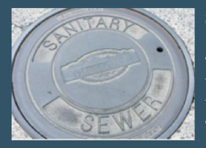
**Sanitary Sewers** collect wastewater from indoor plumbing such as toilets, sinks, washing machines, and other drains and take it to a wastewater treatment plant. The treatment plant removes pollutants from wastewater before it is discharged to the river.
