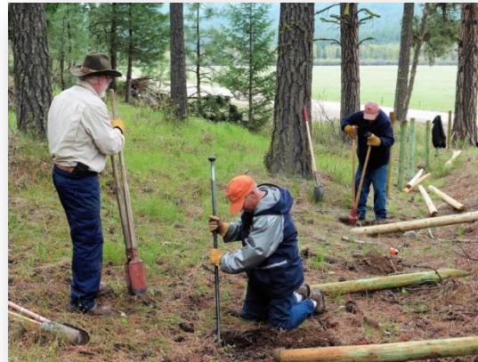
Volunteers installing fencing in Nine Mile
